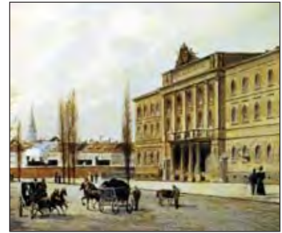
The Austrian Mint, founded in 1194, has been located opposite Vienna's largest public park since 1837.
