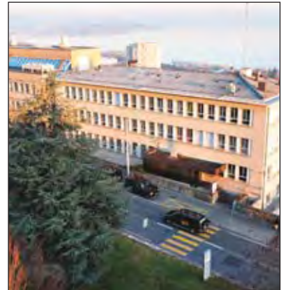
The international headquarters of the Metalor Group in Neuchâtel.
